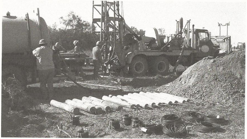
EnvirAnode® installation using familiar drilling, mixing and pumping tools and techniques
