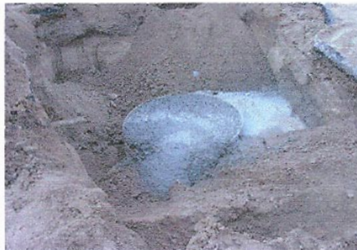
Harcros Well # 6 - Sona-Tube Form filled with concrete prior to backfill.
