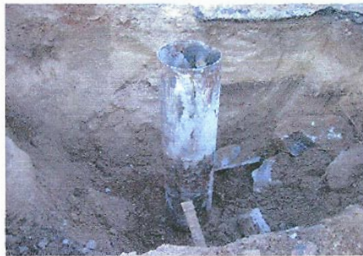
Harcros Well # 6 - exposed 18" well casing after removing pump and prior to cutting casing
