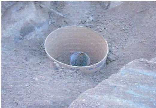
Harcros Well # 6 - Sona-Tube Form over top of cut off well casing. Neat cement placed in well at this time.
