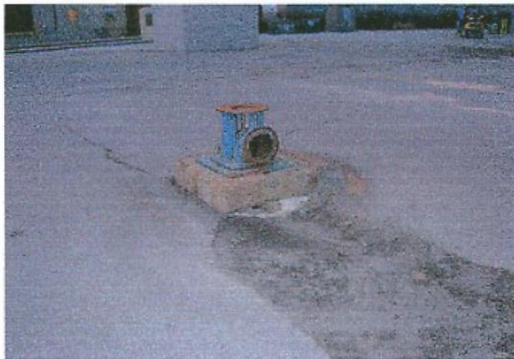
Harcros South Well # 6 - Pump pedestal and concrete base prior to well plugging activities
