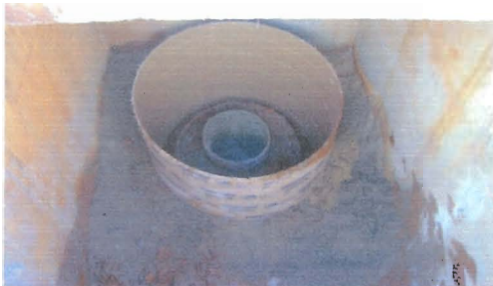
Harcros Well # 5 - Sona-Tube Form over top of well. Note, neat cement in well.
