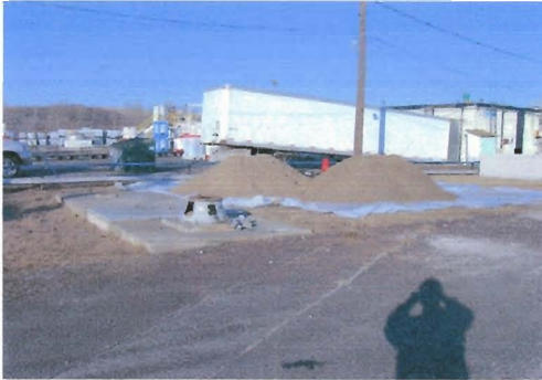
Harcros North Well # 5 - Pump pedestal and concrete meter vault prior to well plugging activities
