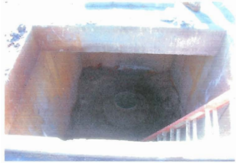
Harcros Well # 5 - exposed 18" well casing and 36" steel outer casing pipe inside meter vault.
