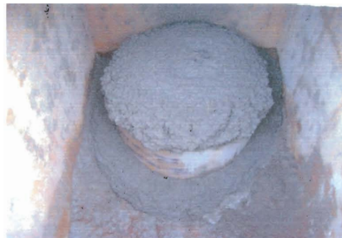
Harcros Well # 5 - Sona-Tube Form filled with concrete prior to demolishing vault and backfill.
