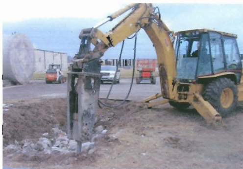
Harcros Well # 5 - demolishing well vault prior to final backfill
