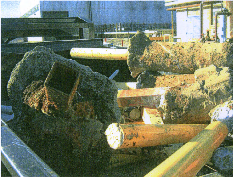
Photograph 37 – Solid debris from well plugging activities. J. Knightly, 1/17/14.
