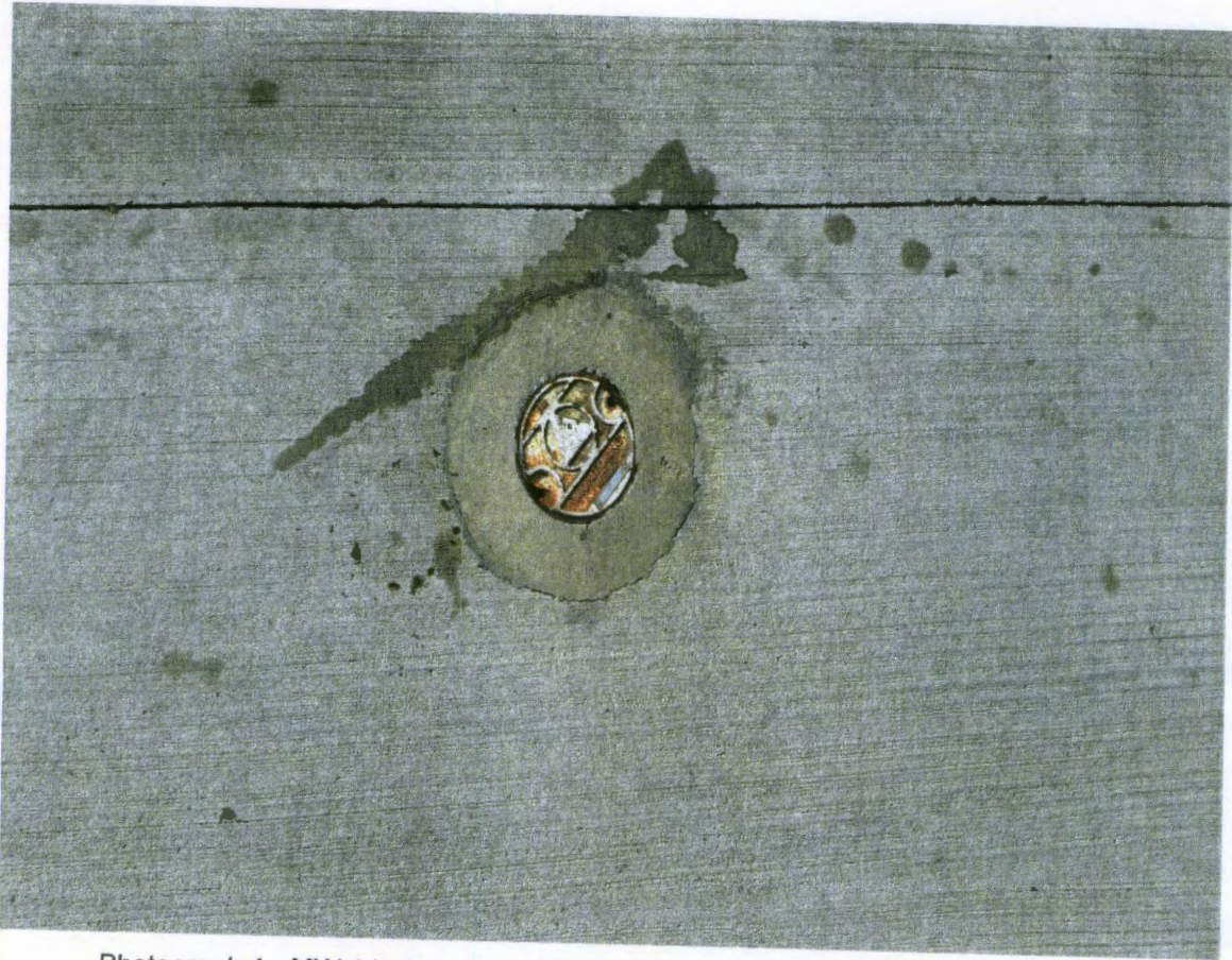
Photograph 1 - MW-1 before plugging. 9/25/15, J. Knightly.
