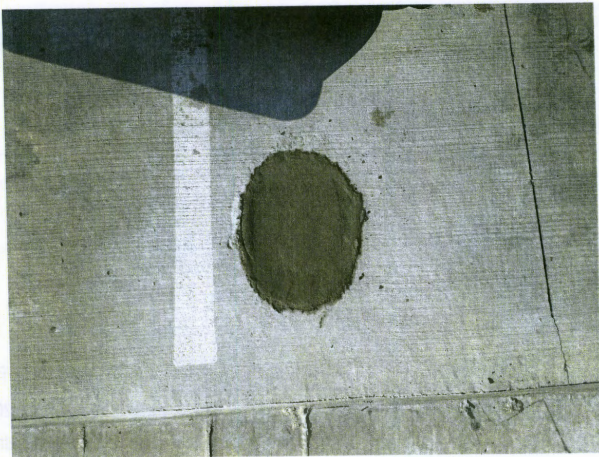
Photograph 4 - MW-2 post plugging. 9/25/15, J. Knightly.
