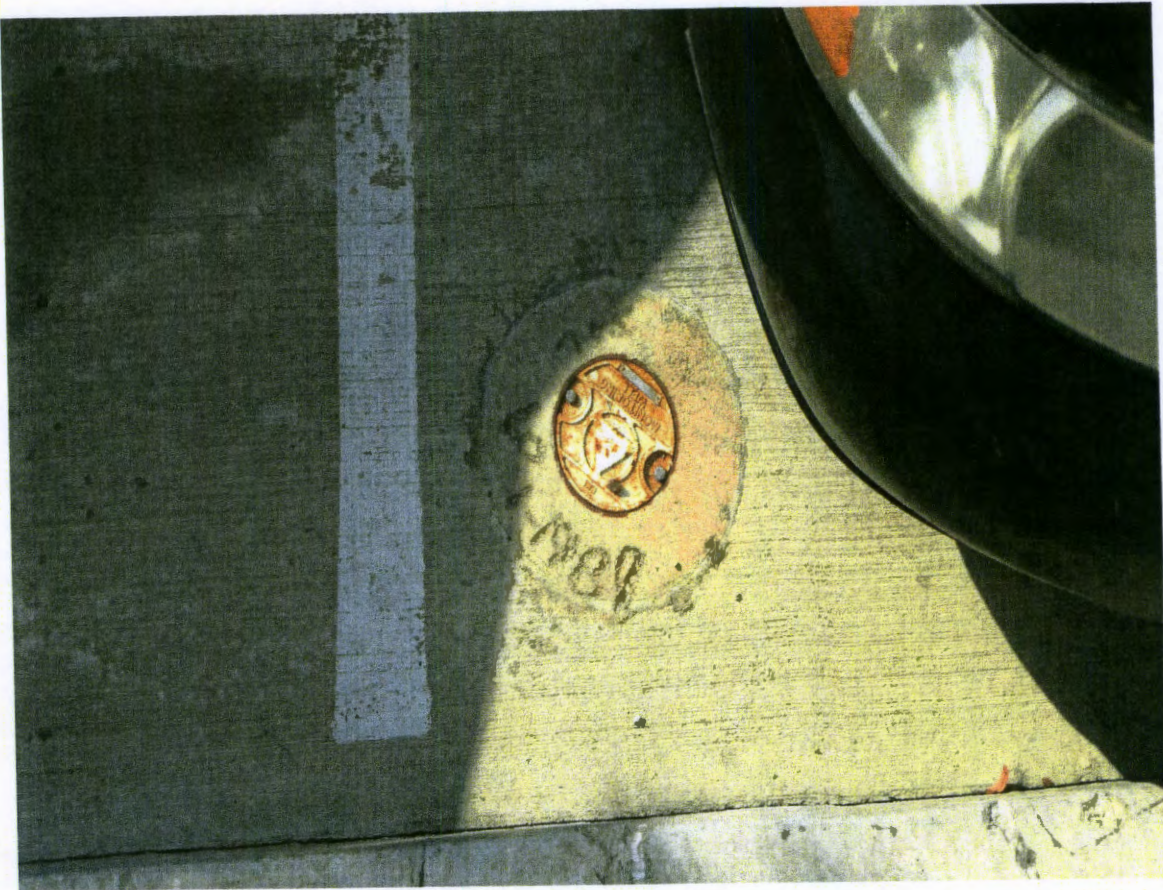
Photograph 3 - MW-2 before plugging. 9/25/15, J. Knightly.
