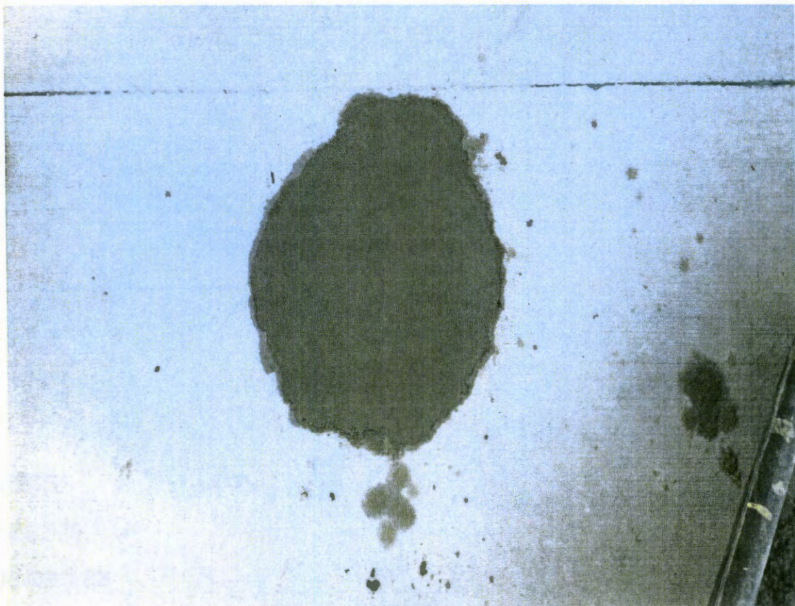
Photograph 6 - MW-3 post plugging. 9/25/15, J. Knightly.
