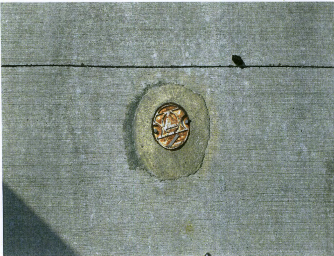
Photograph 5 - MW-3 before plugging. 9/25/15, J. Knightly.
