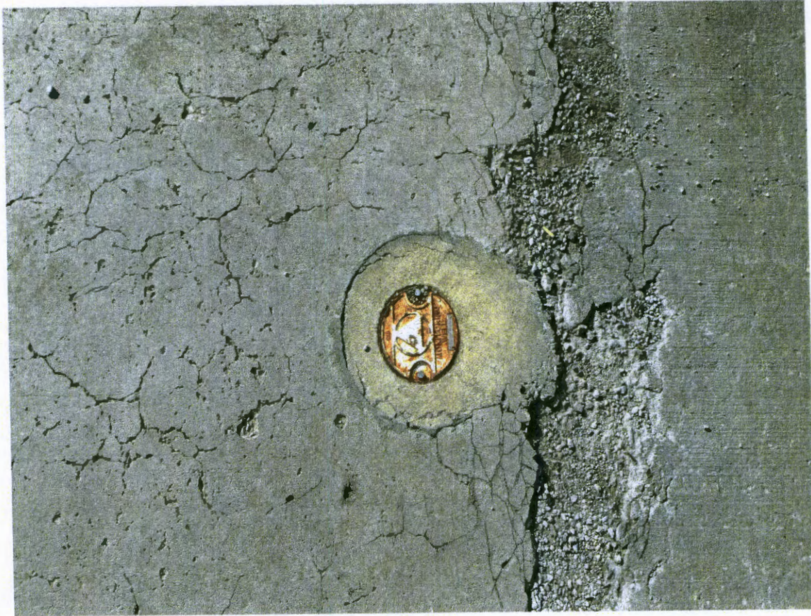
Photograph 7 - MW-4 before plugging. 9/25/15, J. Knightly.
