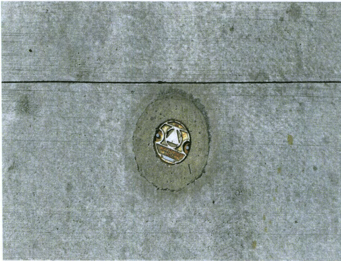
Photograph 9 - MW-5 before plugging. 9/25/15, J. Knightly.
