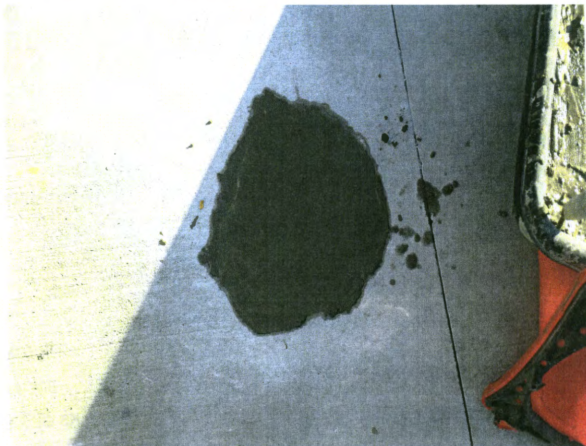
Photograph 12 - MW-6 post plugging. 9/25/15, J. Knightly.
