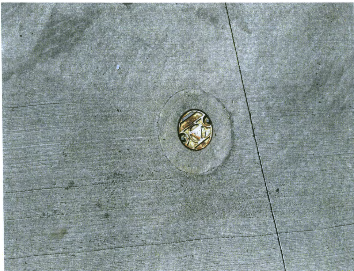
Photograph 11 - MW-6 before plugging. 9/25/15, J. Knightly.
