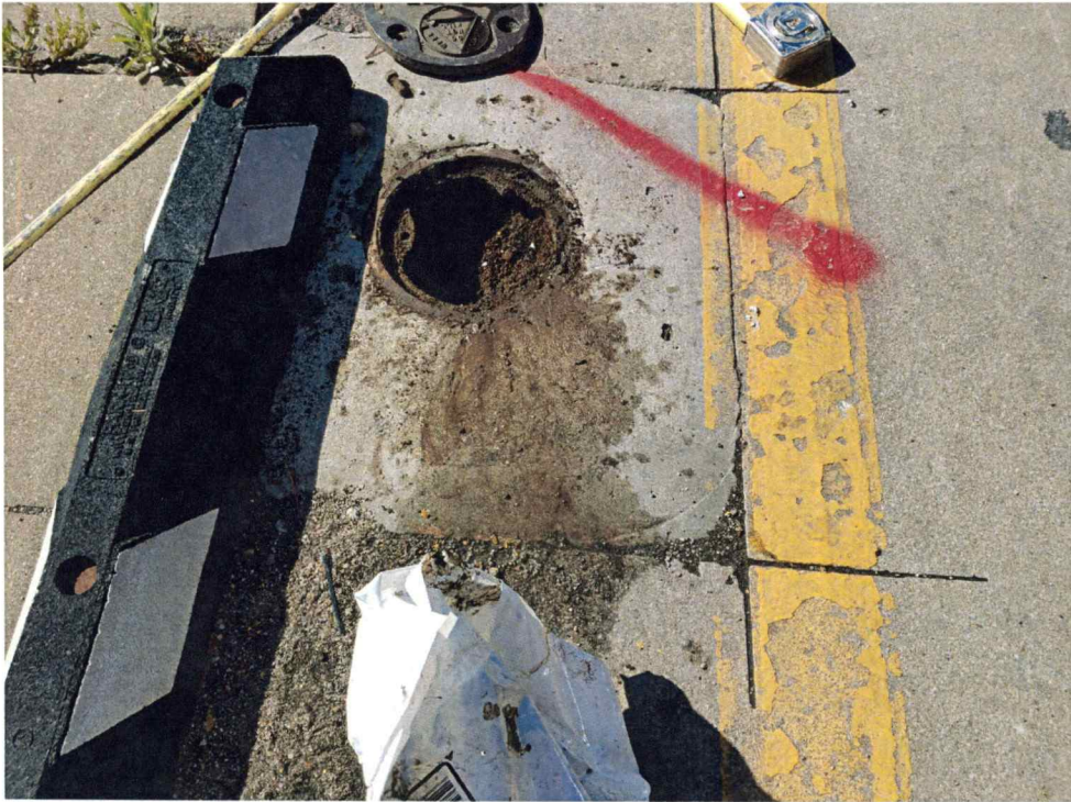
Photograph 9 – MW-8, post plugging. J. Knightly, 04/23/20.
