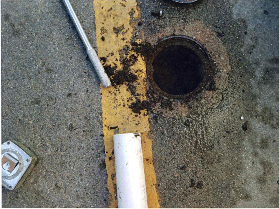
Photograph 5 – MW-4, post plugging. J. Knightly, 04/23/20.
