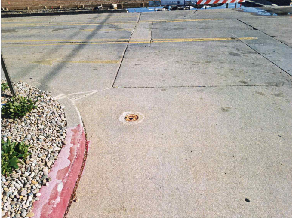
Photograph 6 – MW-6, Pre-plugging. J. Knightly, 04/23/20.
