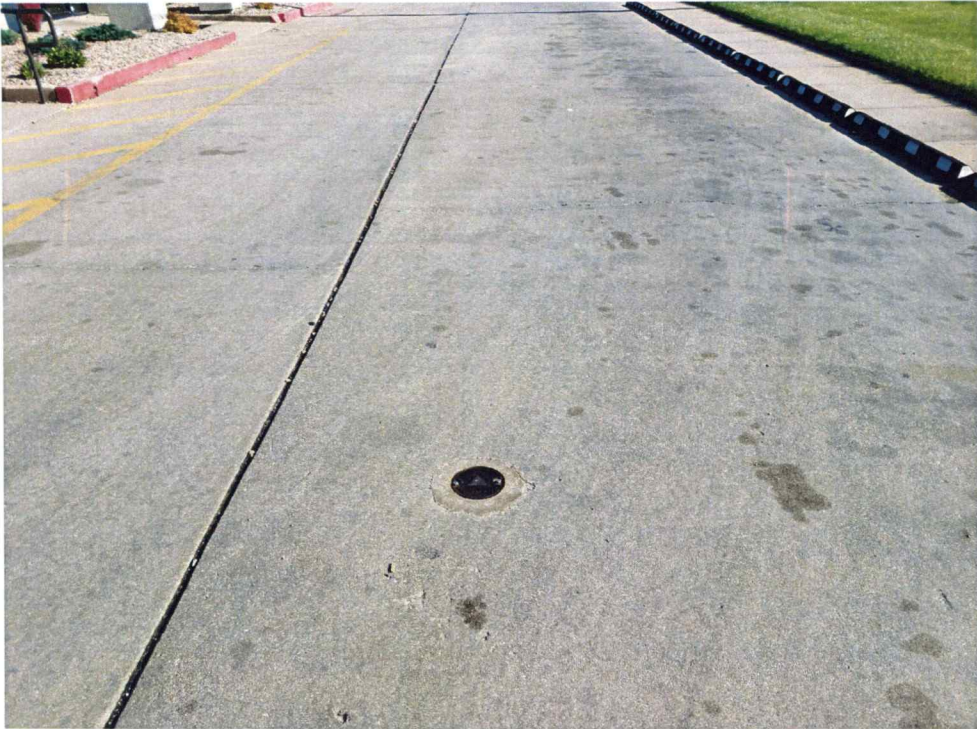
Photograph 1 - MW-3, Pre-plugging. J. Knightly, 04/23/20.
