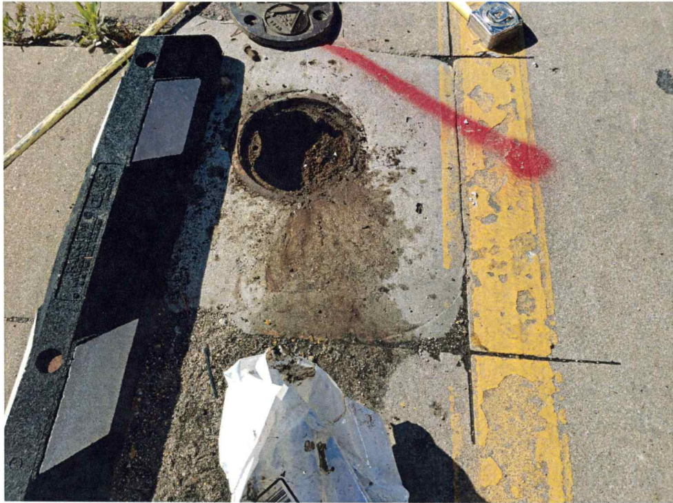
Photograph 9 – MW-8, post plugging. J. Knightly, 04/23/20.
