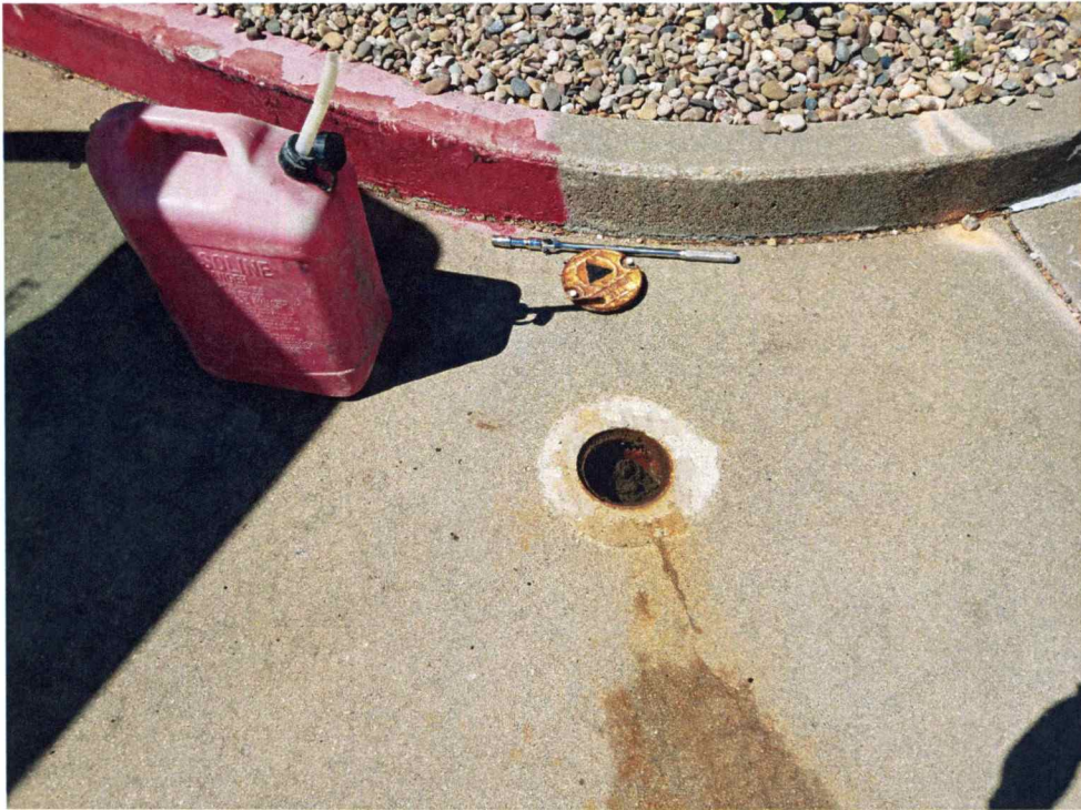
Photograph 7 – MW-6, post plugging. J. Knightly, 04/23/20.
