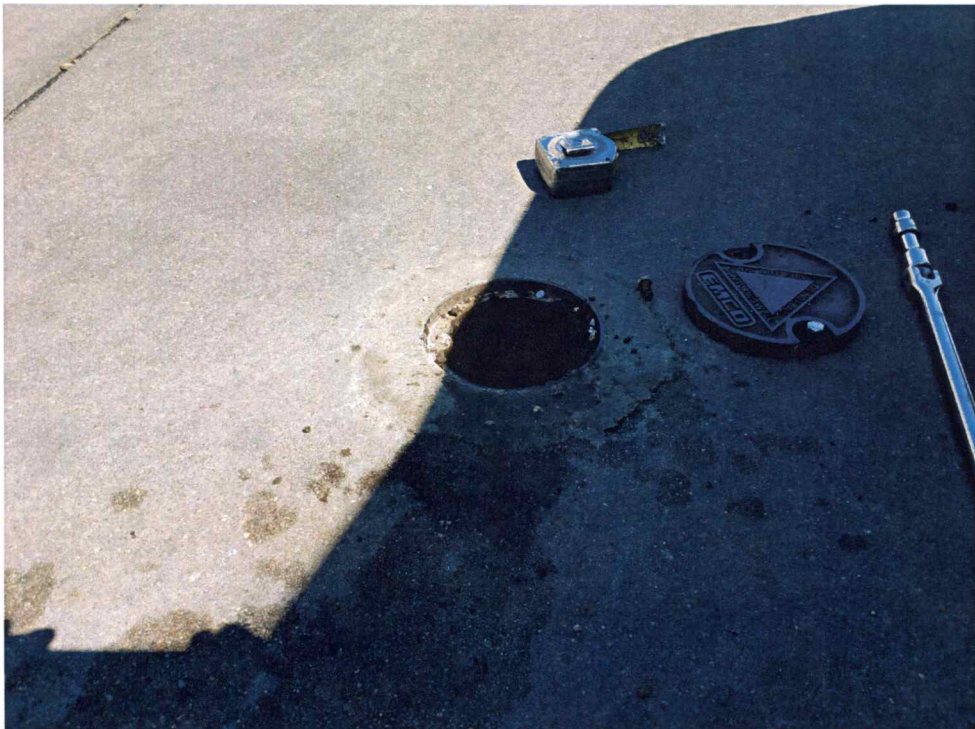
Photograph 2 - MW-3, Post-plugging. J. Knightly, 04/23/20.
