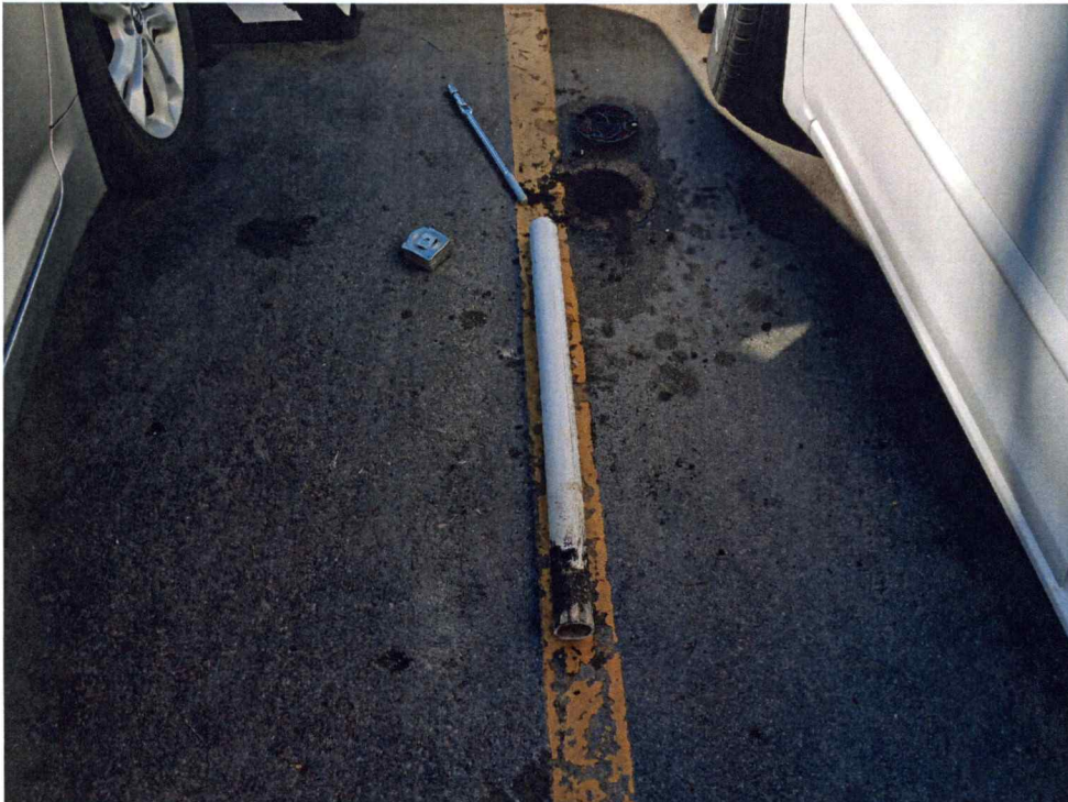
Photograph 4 – MW-4 during plugging. J. Knightly, 04/23/20.
