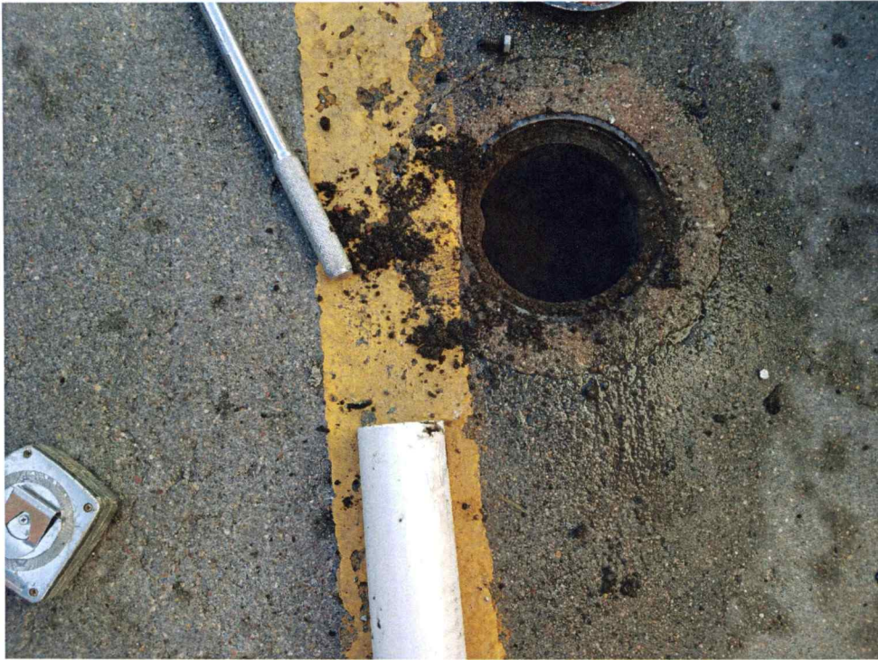
Photograph 5 – MW-4, post plugging. J. Knightly, 04/23/20.
