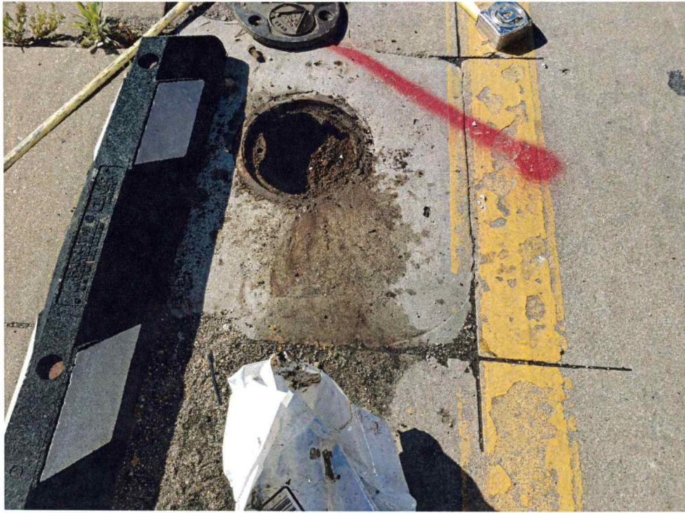
Photograph 9 – MW-8, post plugging. J. Knightly, 04/23/20.
