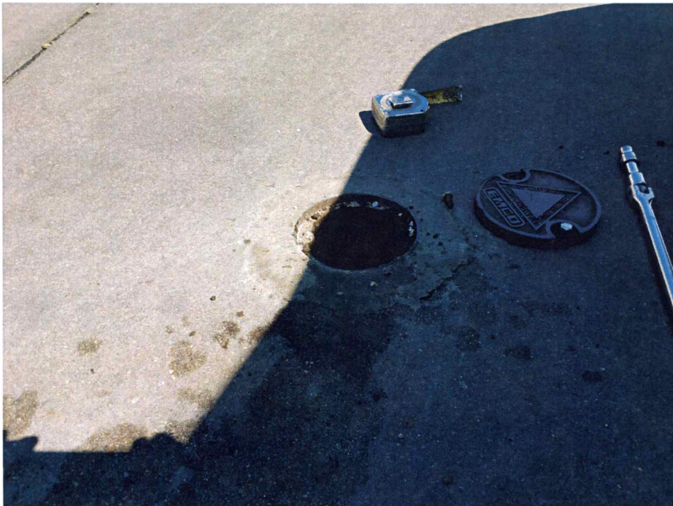
Photograph 2 – MW-3, Post-plugging. J. Knightly, 04/23/20.
