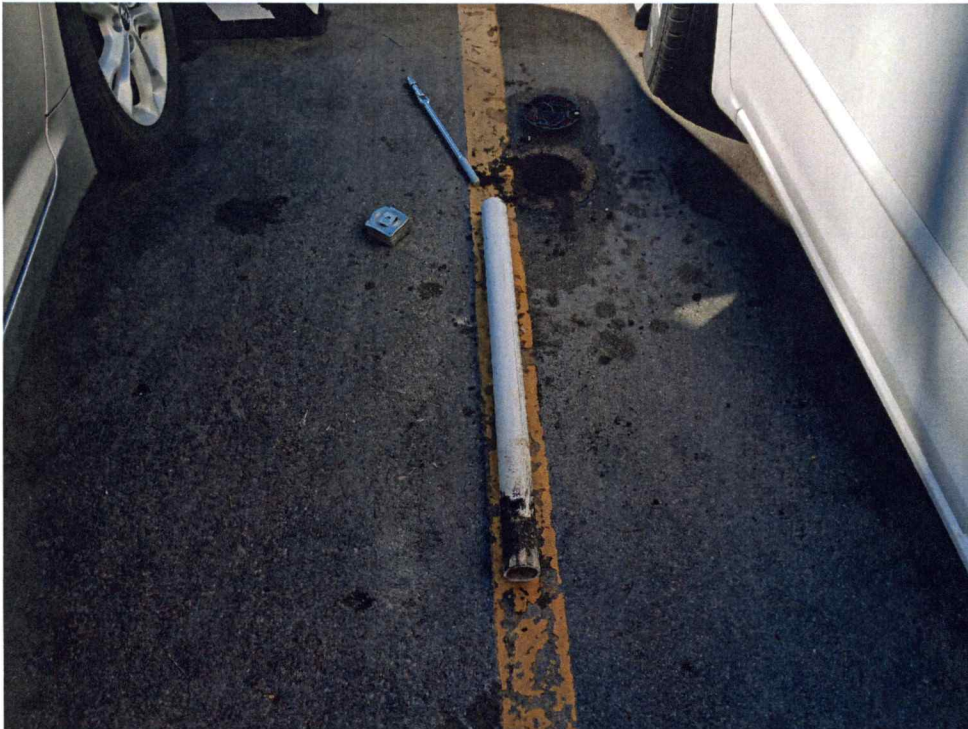
Photograph 4 – MW-4 during plugging. J. Knightly, 04/23/20.
