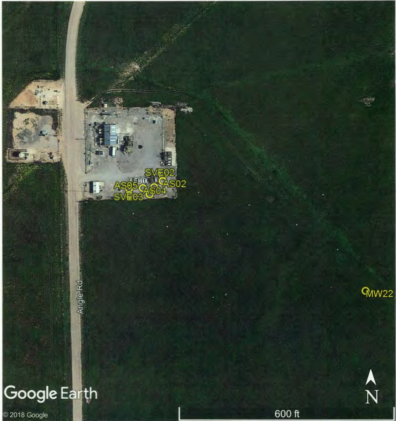
ALL INSTALLED WELLS (Sheet 1 of 2)
